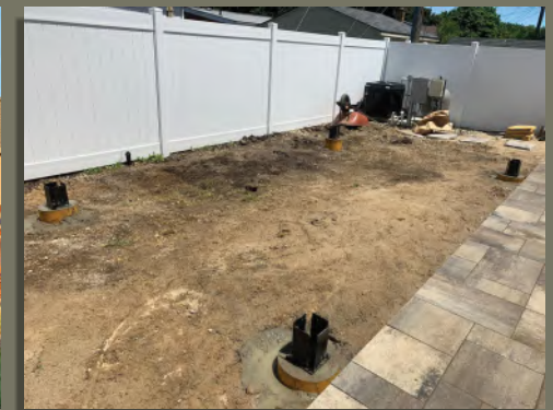
High wind anchors installed in footings
