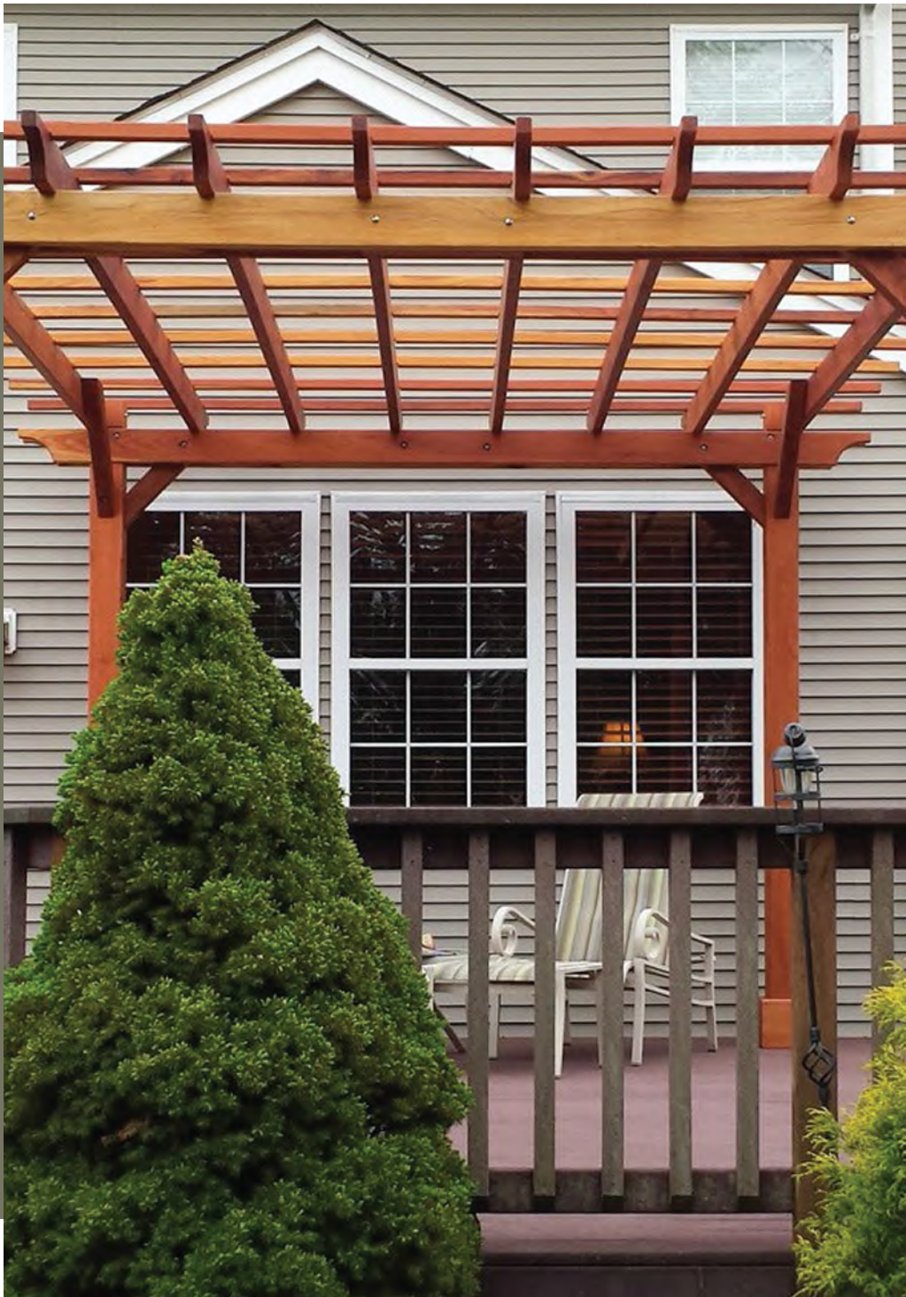
15' x 12' Traditional Garden Pergola with open roof with slats and rafters at 18" and widthwise roof support timbers
