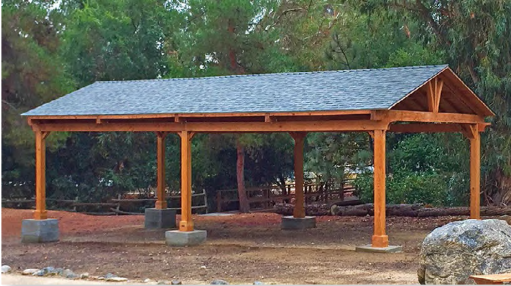
Del Norte Pavilion with a typical asphalt shingled roof.
