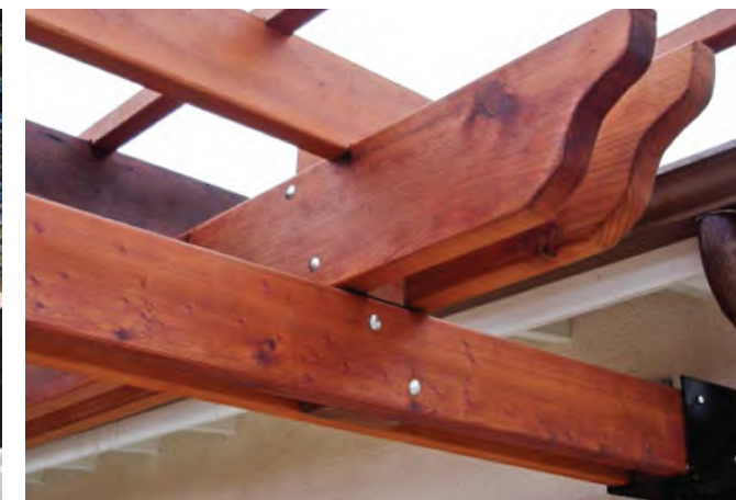
Extensive notching and finishing work
