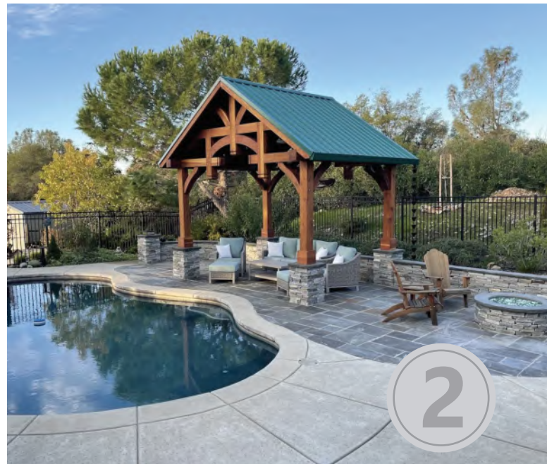
STEVE MOORE SHINGLE SPRINGS, CALIFORNIA THE CARDINAL'S NEST PAVILION Outdoor living room.
