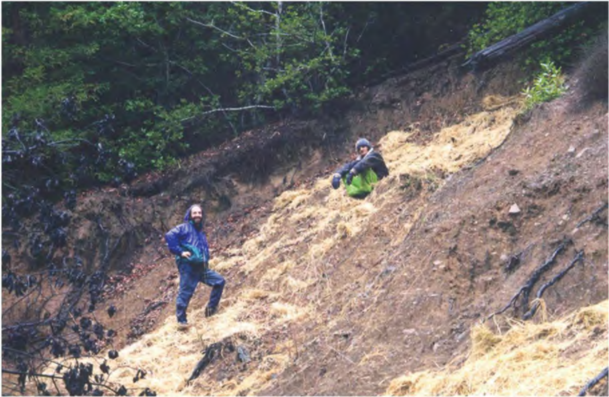
Landslide erosion control: mulching bare soil with sterile hay, Terry Patten and Raul, 1997. (Photo: Jason Johnson)
