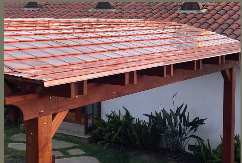
Backyard Pavilion with copper roof
