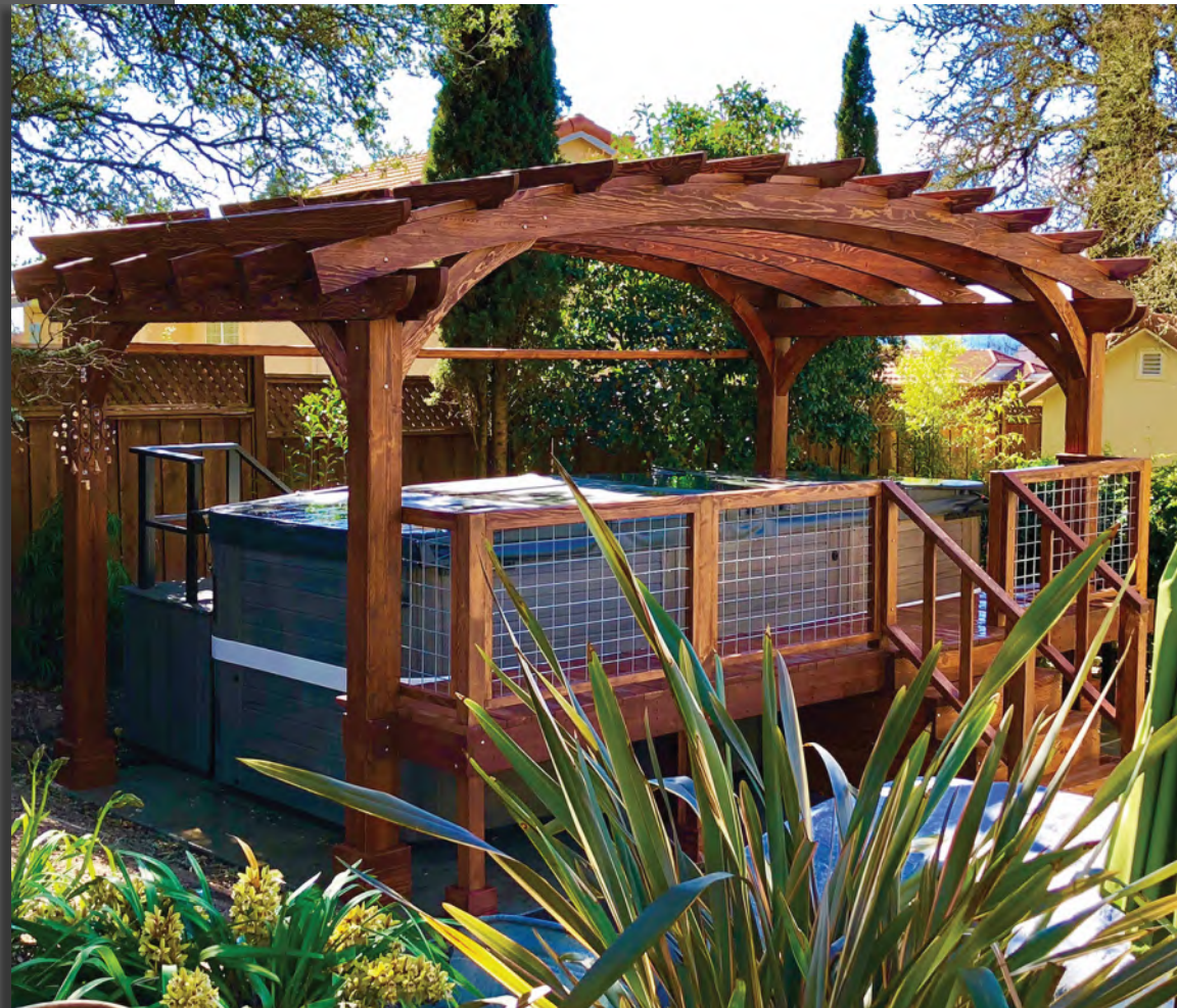
12' x 22' Custom Arched Pergola in Douglas-fir with Coffee-Stain Premium Sealant. Deck and stairs added by custom request. Photo Courtesy of Steve and Heidi J. of Windsor, CA.
