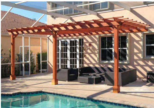
Attached Garden Pergolas (2 photos above) with rafter and slat spacing at 18" on center
