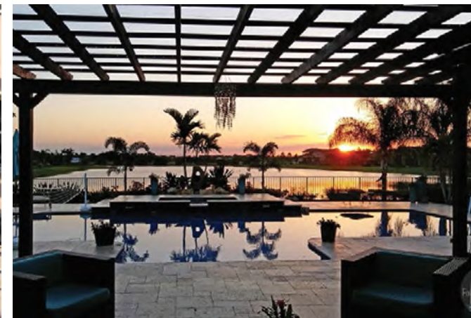
Attached Garden Pergolas (2 photos above) with rafter and slat spacing at 18" on center
