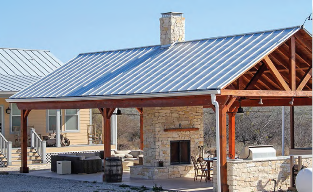
Del Rio Pavilion with a standing seam metal roof.
