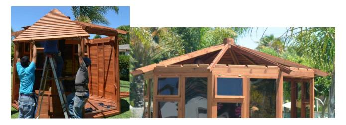
**STEP 7:** Insert the top decoration into the small center base and then continue attaching the rest of roof panels.
