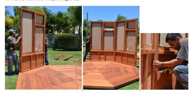
**STEP 3:** Attach the door frame to the wall panels with deck screws 3" x #8.
