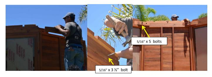
**STEP 5:** Attach the rafters to the roof base and small center base with bolts washers & nuts. (Match up the numbers to attach the two parts together). Tap the bolt all the way into the wood to set it. Then add a washer and nut and lightly tighten.
