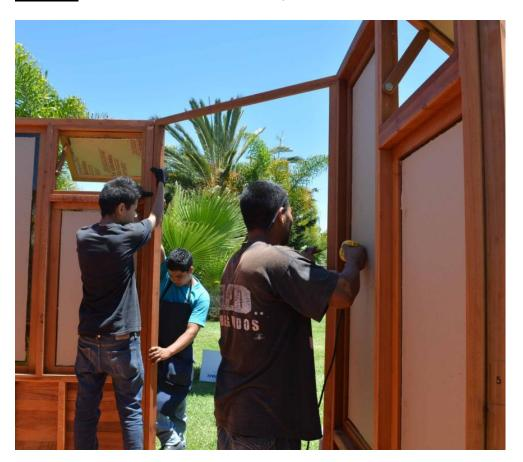
**STEP 4:** Attach the timbers together to form the base of the roof with bolts, washers & nuts. (Match up the numbers to attach the two parts together). Tap the bolt all the way into the wood to set it. Then add a washer and nut and lightly tighten.
