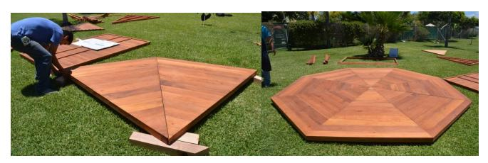
**STEP 2:** Attach the wall panel to the other wall panel and floor with deck screws (3"x #8). (Match up the numbers to attach the two parts together).
