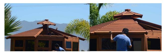
**STEP 8.** Attach the roof trims between each roof panel, atop the rafters, with three deck screws (3"x #8). Fill any gap with silicone.
