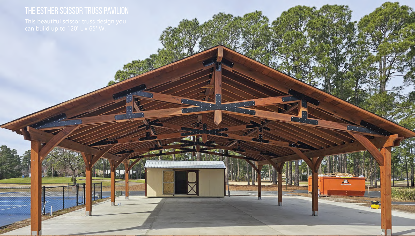
Photo shows the interior roof boards of a Esther Scissor Truss Pavilion in California Redwood.
