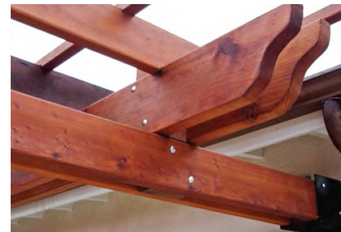
Extensive notching and finishing work
