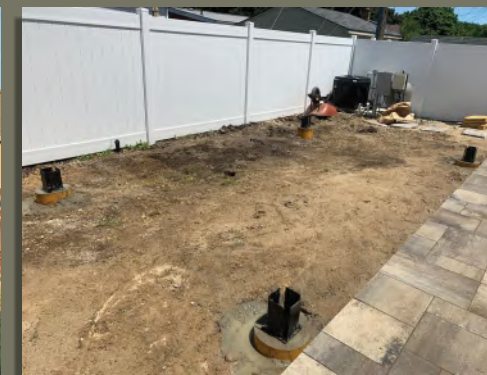
High wind anchors installed in footings
