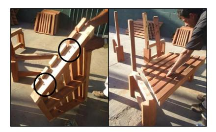
**Step 2:** Attach the front pieces the seat & the leg with four bolts (5/16" x 4"), washers and nuts.
