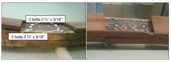
**2** Attach part C (joint cover) to part A (arc), with four deck screws (2" x 6"), washers & nuts (into four holes marched "2"). Repeat in the other side.
