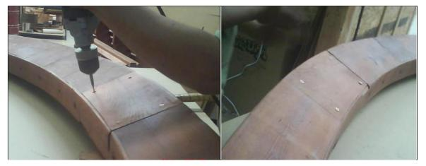
**3** Attach part E (leg) to part A (arc), with bolt (9" x 3/8"), washer & nut (into hole marched "4"). Tap the bolt all the way into the wood to set it. Then add a washer and nut and lightly tighten. Repeat the other size.
