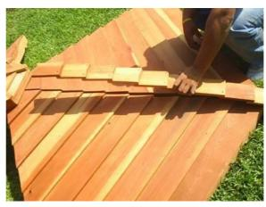
**Photos 13, 14**: To complete the roof, long strips with triangular ends are set with screws on the joints of the roof, as picture 13 and 14 show.
