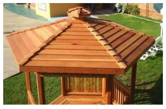
**Photos 11, 12**: Picture 11shows how each section of the roof is being assembled with two bolts, side to side. On the top there will be a crown that will also help to hold the upper part of the roof, as shown in picture 12. The roof can be fully assembled before is set on top, or installed section by section until it is completed.
