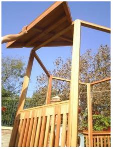
**Photos 9,10**: Photos 9 and 10 show the next step, put each one of the triangles over each wall (Section C). Over the top cross support on each wall there is a mark with the letter C and a number that matches with roof number that will be installed over the cross support; then each part of the roof is installed until the roof is finished.
