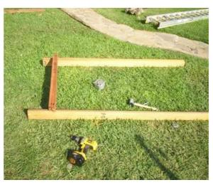
**Photo 3**: Start by building the main wall, this is the door frame of the gazebo.
