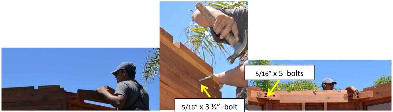
**STEP 5:** Attach the rafters to the roof base and small center base with bolts washers & nuts. (Match up the numbers to attach the two parts together). Tap the bolt all the way into the wood to set it. Then add a washer and nut and lightly tighten.
