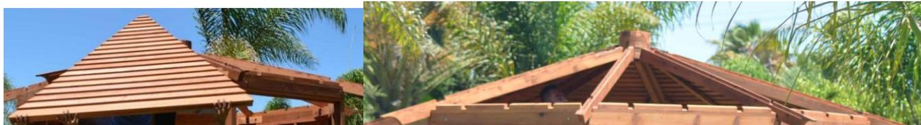
**STEP 7:** Insert the cupula in the small center base and then continue putting the rest of roof panels.
