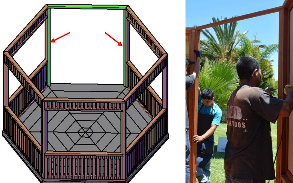
**STEP 4:** Attach the timbers together to form the base of the roof with bolts, washers & nuts. (Match up the numbers to attach the two parts together). Tap the bolt all the way into the wood to set it. Then add a washer and nut and lightly tighten.
