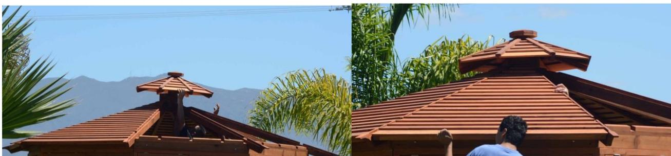
**STEP 8.** Attach the roof trim between each roof panel with three deck screws (3"x #8). And repeat the process for each space between the installed roof panels and fill between gaps with silicone.
