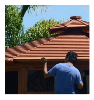
**STEP 7.** Attach the roof trim between each roof panel with three deck screws (3"x #8). And repeat the process for each space between the installed roof panels and fill between gaps with silicone.
