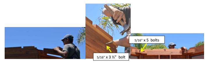
**STEP 5:** Attach the rafters to the roof base and small center base with bolts washers & nuts. (Match up the numbers to attach the two parts together). Tap the bolt all the way into the wood to set it. Then add a washer and nut and lightly tighten.
