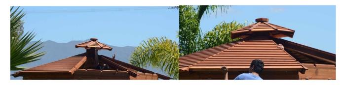
**STEP 8.** Attach the roof trim between each roof panel with three deck screws (3"x #8). And repeat the process for each space between the installed roof panels and fill between gaps with silicone.
