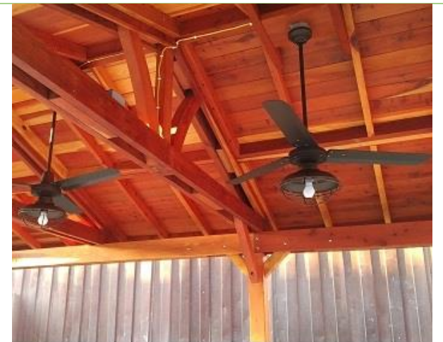
Pavilion with 2 Ceiling Fan Base
