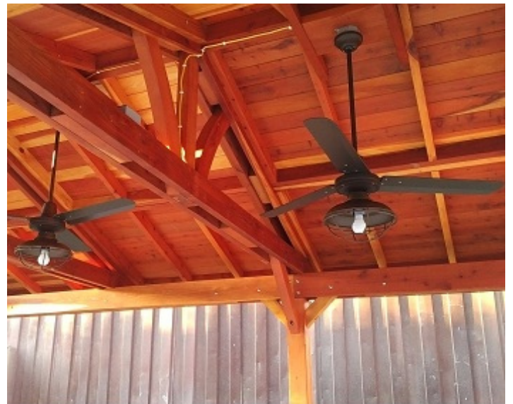
Pavilion with 2 Ceiling Fan Bases
