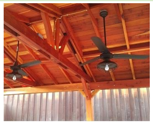
Pavilion with 2 Ceiling Fan Base
