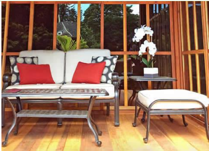
Interior Decking (2" X 6" boards with 1/32" separation between the boards).
