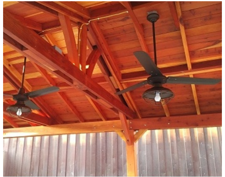
Pavilion with 2 Ceiling Fan Bases
