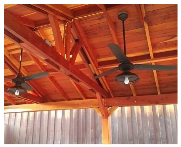
Pavilion with 2 Ceiling Fan Base
