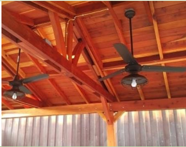
Pavilion with 2 Ceiling Fan Bases
