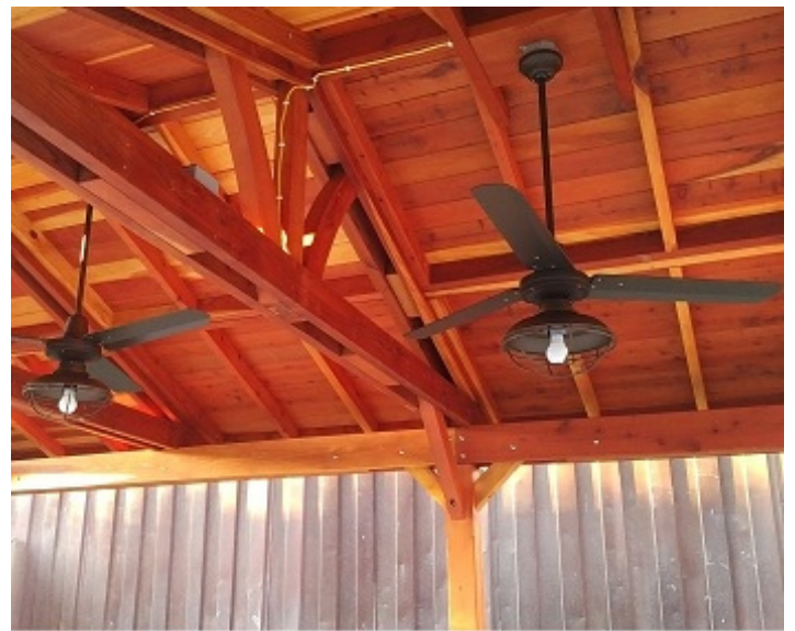
Pavilion with 2 Ceiling Fan Bases
