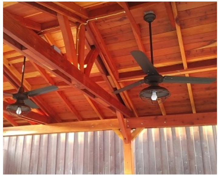
Pavilion with 2 Ceiling Fan Bases
